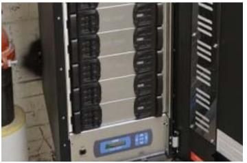
now and well into the future. By utilizing the modular design to deliver all phases of power to single pole, double pole, and dimming devices, the hybrid nature of PCS TRIO™ was the answer for their needs. Being in the final stages of the project other key factors that appealed to SWA included the availability of stock and simplicity of installation that PCS TRIO™ offered.
